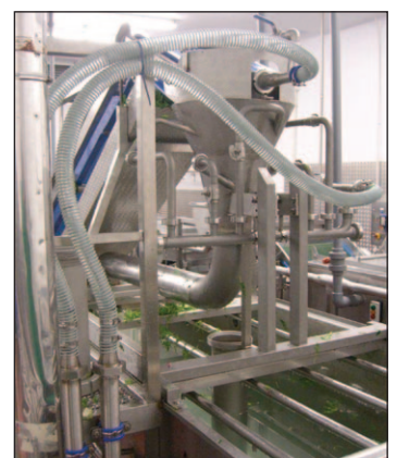
Air and water pipework
