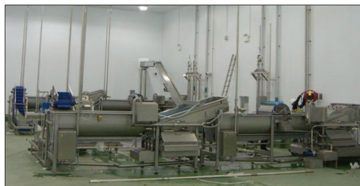
Equipment positioning, installation & connection
