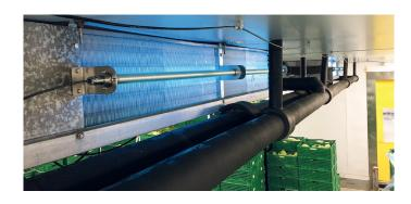
sterilAir® offers a powerful and environmentally friendly solution. Our UVC installations sustainably prevent build up and growth of biofilm. Clean coils keep the energy consumption of the cooling unit constantly low. The slats remain hygienically flawless, cleaning effort and frequency decrease significantly - a considerable cost saving in operation and maintenance.
